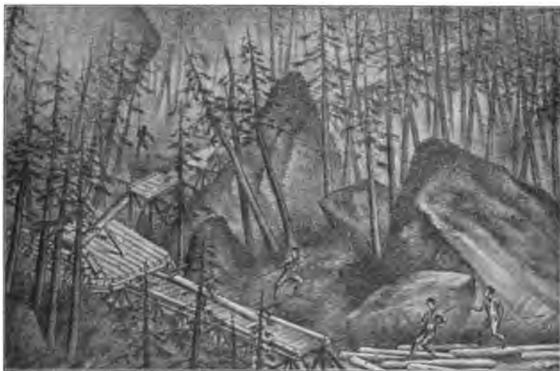
Fig. 206.—Change of direction in Japanese slide. From a Jap. State publication.
